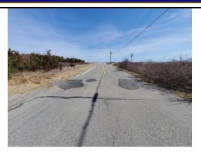
Asphalt and rock patches on Hawes Avenue due to broken culvert pipe under roadway (taken 3-15-2022).
